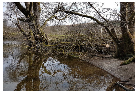
Fig. 2.4 Coppiced tree limes secured into an eroded bank
