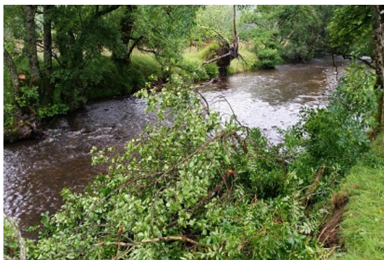
Fig. 2.3 Felled trees secured into the bank
