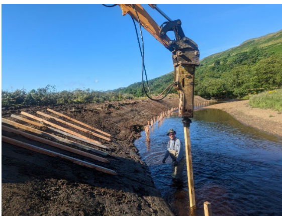
Fig. 2.9 Installing posts along the reprofiled bank face
