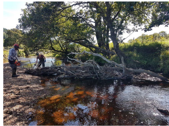
Fig. 2.14 Reducing a woody debris dam
