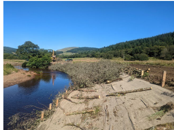
Fig. 2.12 Willow brush and log laid onto the hessian layer
