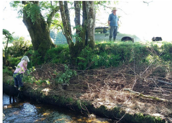
Fig. 2.6 Installing green bank revetment to protect existing trees
