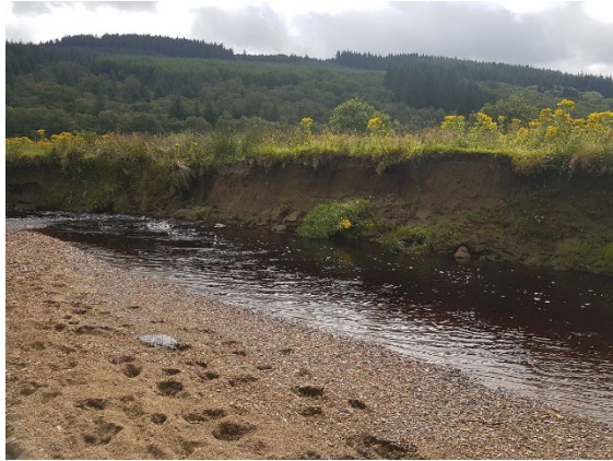
Fig. 2.7 Eroding bank face at treatment site
