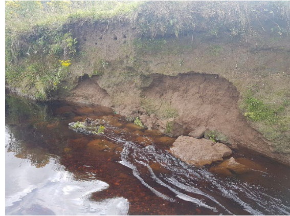
Fig. 2.8 Bank collapse and soil deposits
